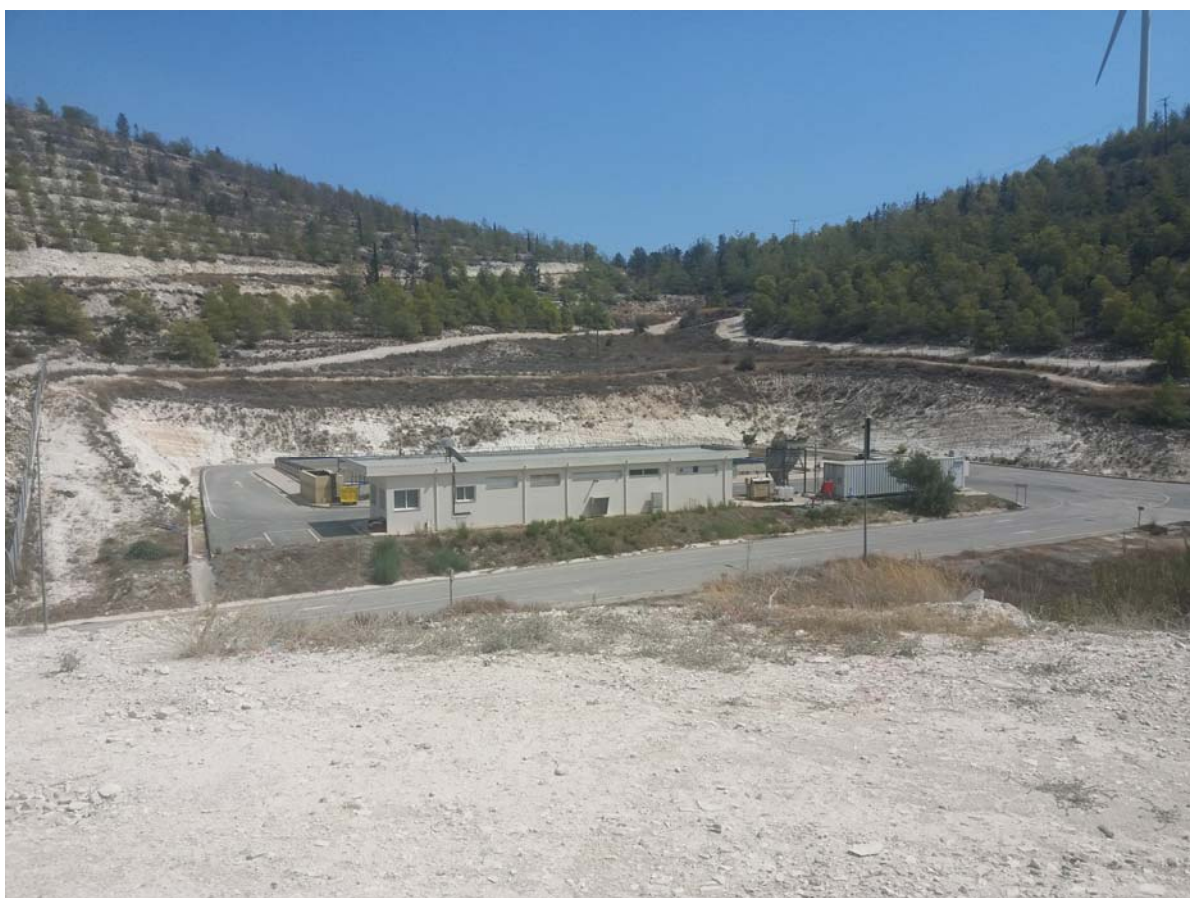
Figure 5: Waste Water Treatment Station
