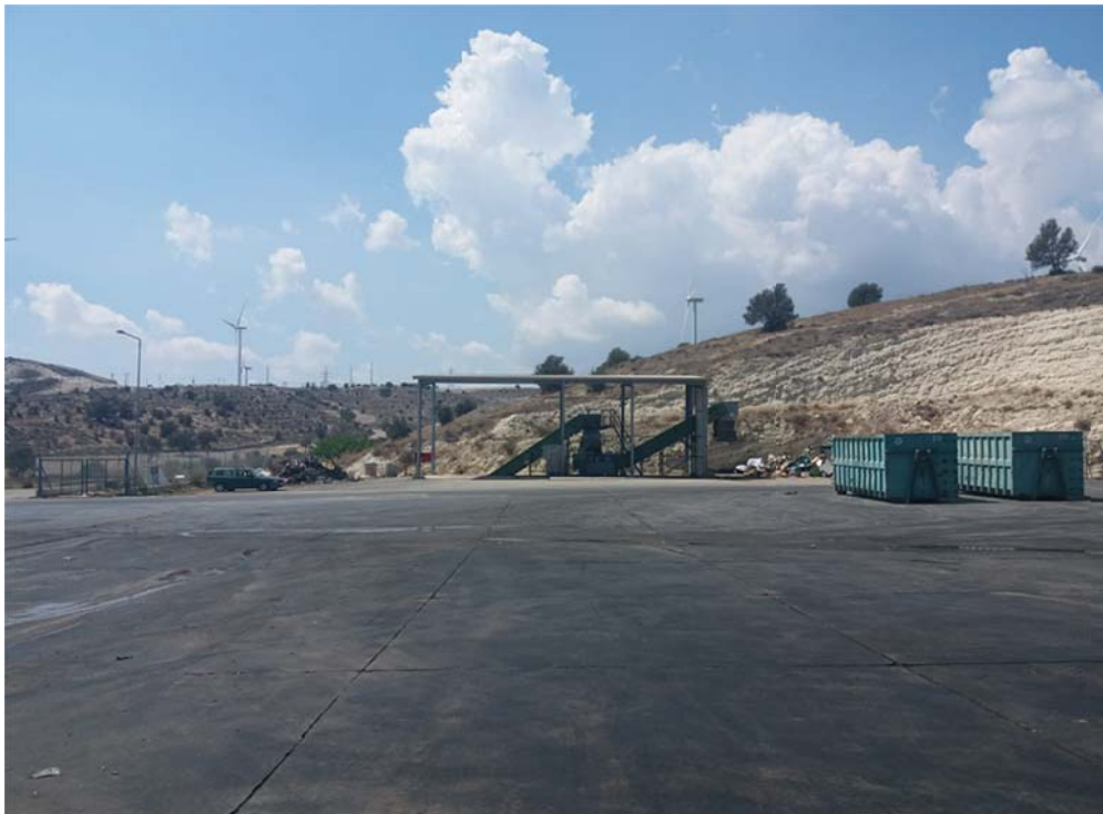
Fig.3: Photo of the inspected solid domestic waste treatment facility in Larnaca-Famagusta Districts
