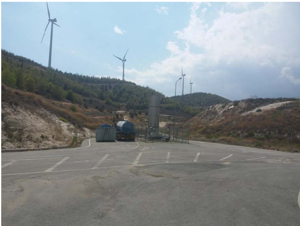
Fig.5: Biogas unit at the inspected site.
