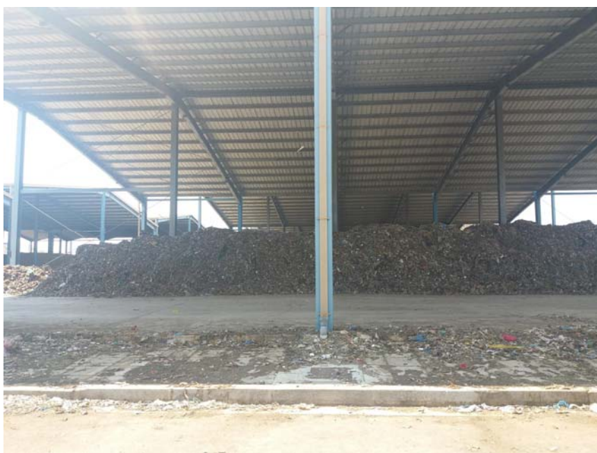
Figure 4b: Composting area
